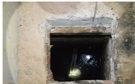
Figure 1: The sheep being down in the septic tank (white color).
